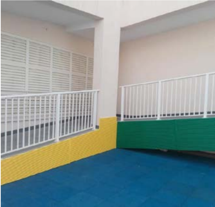
Photos of Wall & Column Padding installed
