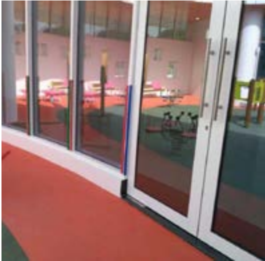
Photos of Corner Guard installed
