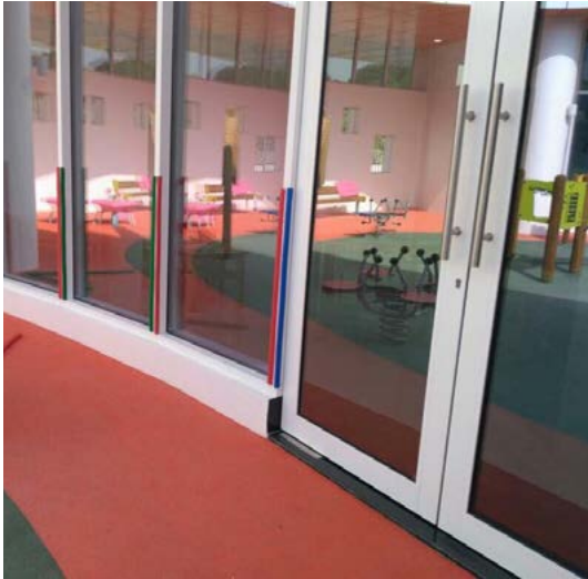
Photos of Corner Guard installed
