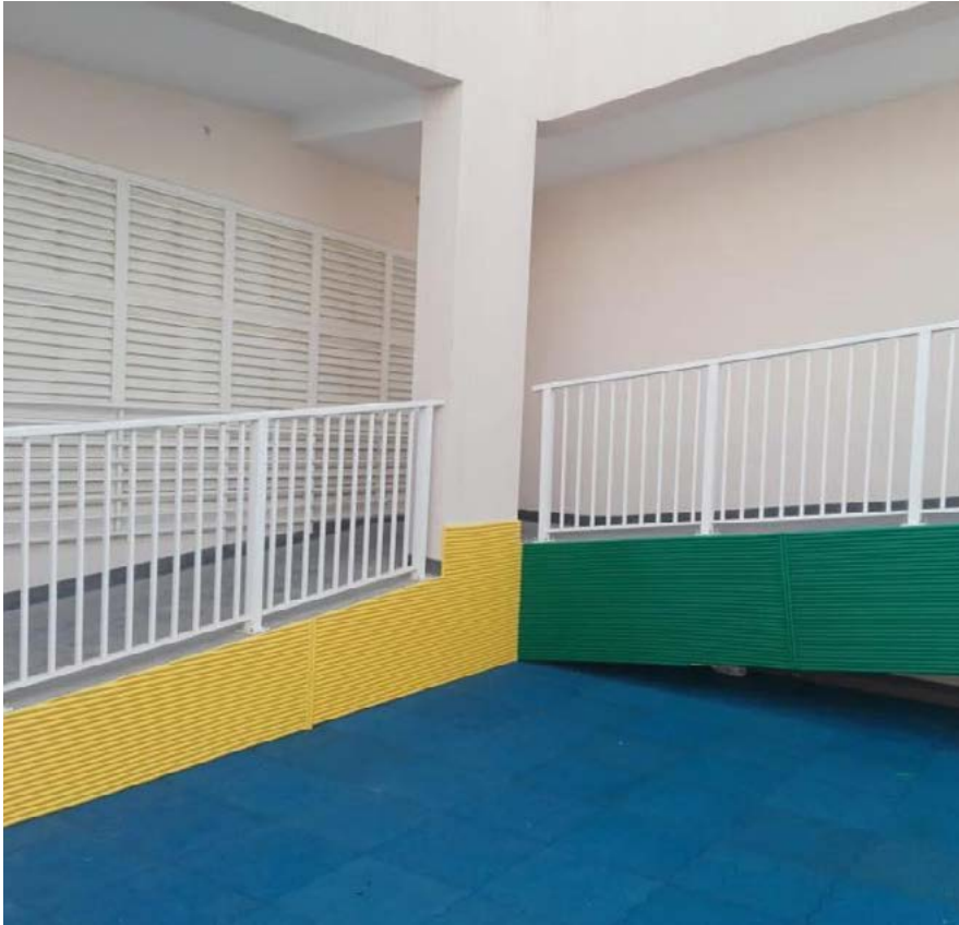
Photos of Wall & Column Padding installed
